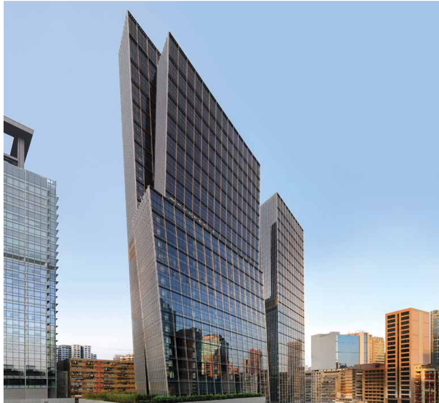
Landmark East Building, Hong Kong
